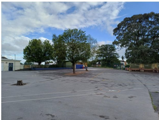
The Lower Playground and the toilets
